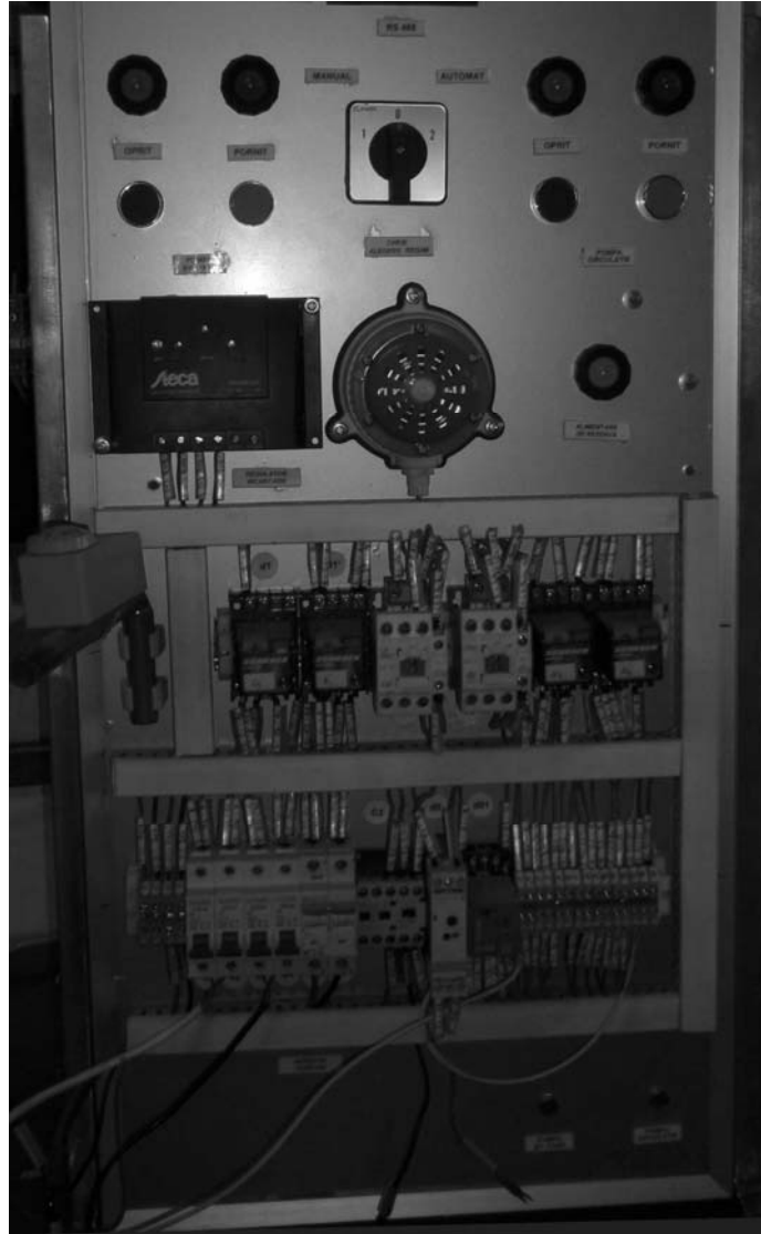
Figure 1 Gasification boiler control system
